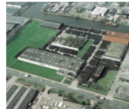
Casing warehouse in Emmeloord.
